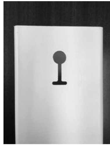
3: Top Keyhole Slot is mirrored upside down from all bottom keyhole slots - gravity and shape of keyhole slot keeps bungee in place
