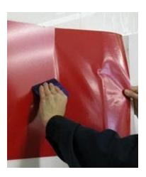
h) Re-squeegee the entire graphic using very firm squeegee pressure, including all edges. Puncture any air bubbles with a straight pin and re-squeegee from the edge of the bubble towards the puncture.
