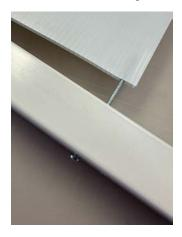
3. The corrugated sign must have the flutes landscape (horizontal). Put the screw into the top slot of the post and fasten into one of the top flutes of the sign. Snug the screw (leave a bit loose so that it slides up & down in the slot).
