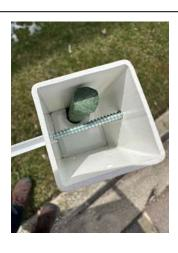
4. There are two stake inserts inside each pvc post. Carefully slide each stake into the top and then bottom inserts. Once you see the stakes coming out of the bottom of the pvc posts you can pound the stakes into the ground. We include a pvc block to place on the top of the stake when it is near the pvc post so your hammer doesn't break the post. The stake should be set below the top of the pvc post so there is room for the cap to be mounted.
